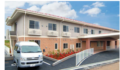
Day Service / Short Stay facility
